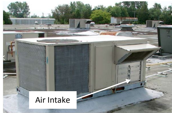
Typical HVAC Unit with Outside Air Intake
